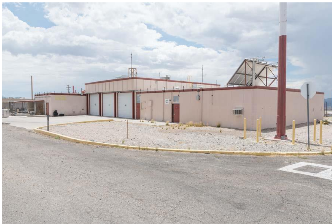
Figure 12-3. The historic Mercury Fire Station, viewed to the southwest at the corner of Buster Street and Sandstone Avenue (RSL 2018)
