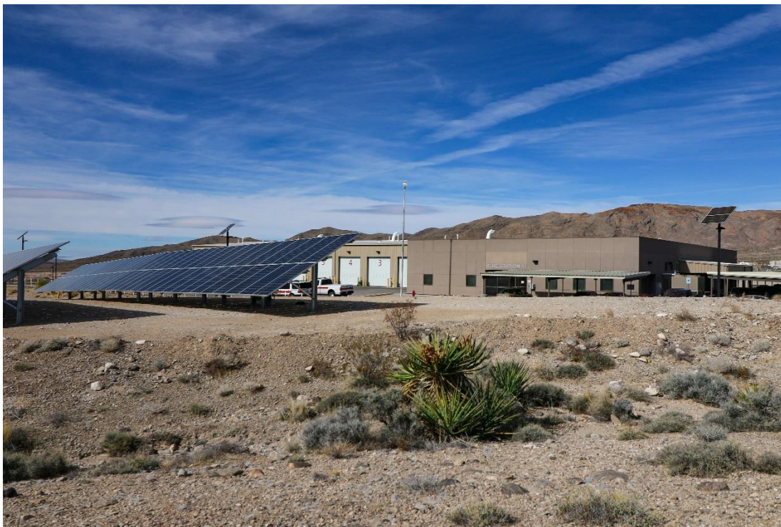
Figure 3-2. Solar PV Demonstration Project at the Mercury Fire Station
