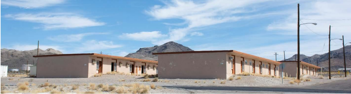
Figure 12-4. View of the 475-479 dormitory complex from Greenhouse Avenue, facing northeast (DRI 2019)
